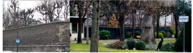
Fig. 2 The wall from outside and inside
